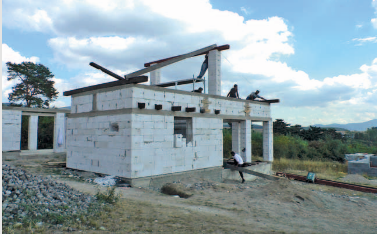
Fig.: Placing the rafter on the wall plate
