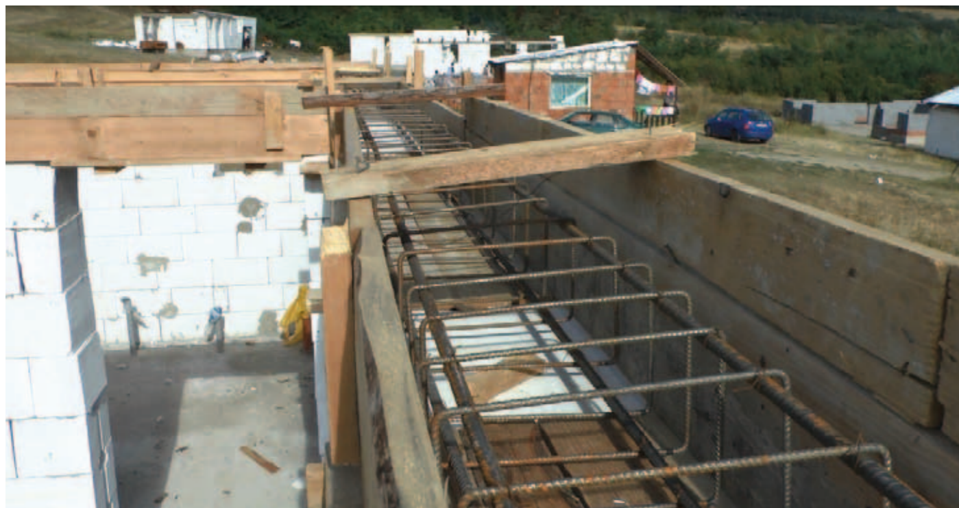
Fig.: Placing the reinforcing steel bars into the bond beam
